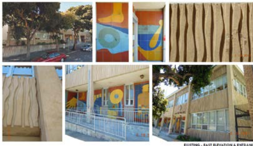
EXISTING - EAST ELEVATION & ENTRANCE
